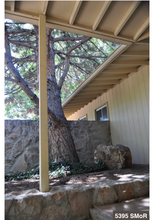
A wood column carries the cantilevered roofline above the entry stairs.
