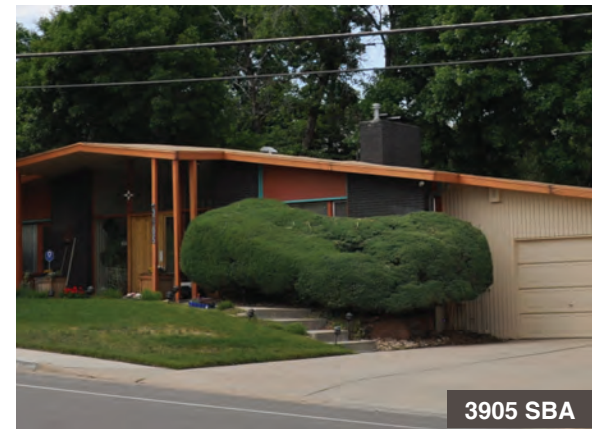
This staircase rises from the front walkway along a masonry planter to the front entrance.
