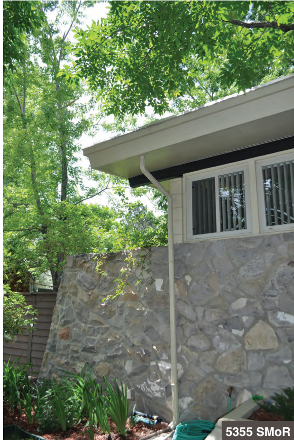
This wall and roof both extend beyond the body of the house. The end of the wall and the fascia of the roof are angled in opposition to each other, enlivening the overall horizontality of the house.
