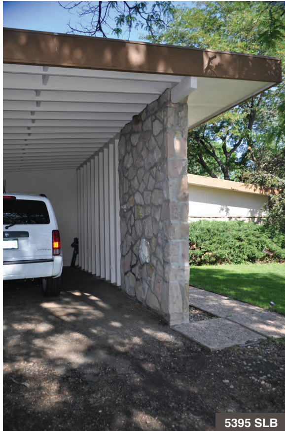
This shed roof extends over the side wall of the carport to shelter the walkway to the front entrance.
