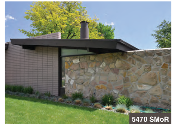
Such walls amplify the scale of the houses. Careful examination is required to see that the house does not extend the full length of the wall, but stops short at the exposed beam above.
