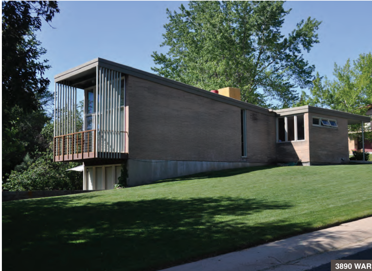
A long shed roof and flat roof are combined on these two, perpendicular volumes.
