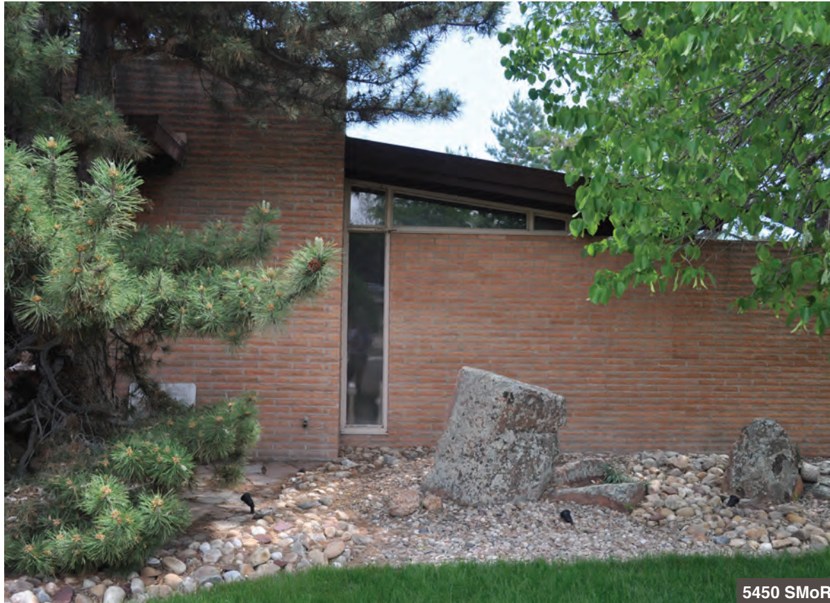
This composition includes a full-height fixed vertical pane that rises to a row of windows below the low-pitch front-gable roof.
