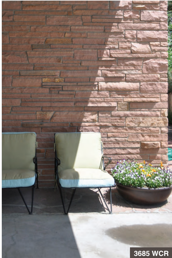
Walls are constructed of random range ashlar masonry, using flat slabs of native red sandstone from the Lyons area. Stones occasionally project beyond the of the wall plane, adding a decorative visual element.
