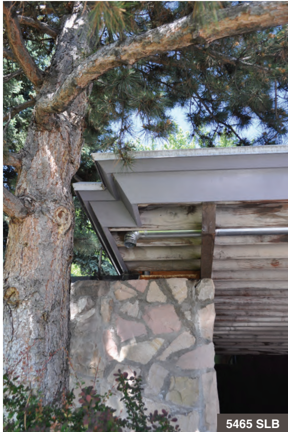
This complex eave detail appears over an open carport. The prominent fascia has two angled facets. It steps back as it turns onto the adjacent elevation, forming an indented corner.
