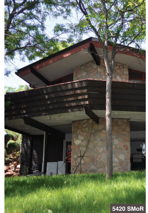
This projecting balcony wraps around three sides of this angled two-story chimney in an east-facing back yard.
