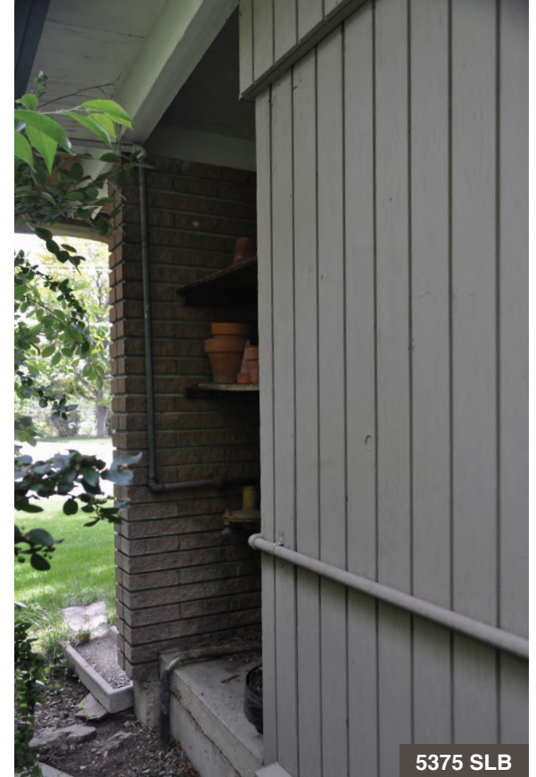
Projecting walls sometimes serve utility purposes as well. This front wall extends beyond a recessed alcove that shelters the water meter.
