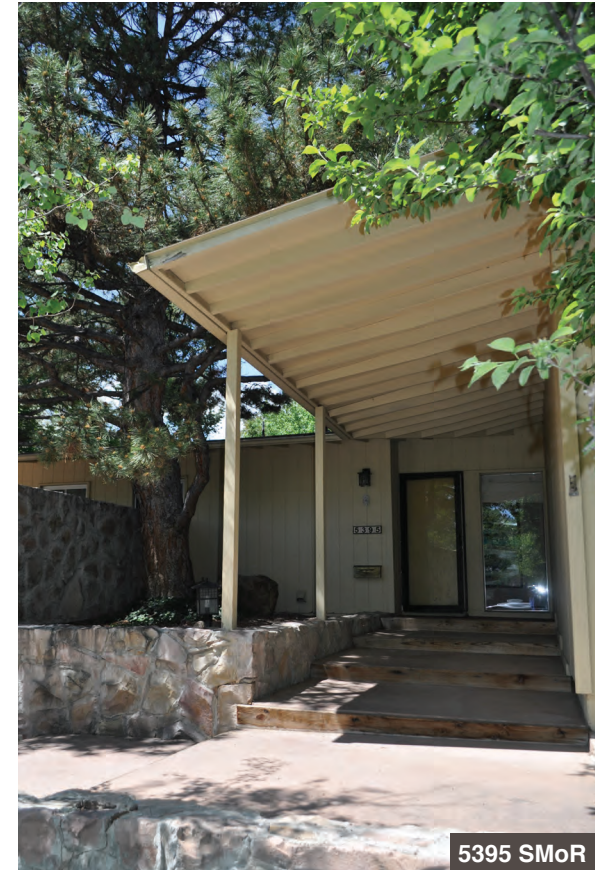
The varied roof planes extend beyond the wall planes to shelter staircases, walkways and entrances, as seen here.
