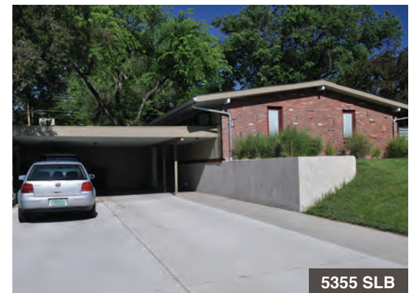
This house features two opposing shed roofs, the top roof extending to overlap the lower roof.
