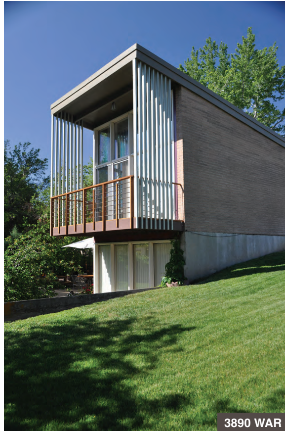
Here the roof, wall and floor planes all project beyond the body of the house to form a semi-enclosed balcony with an eastern view.
