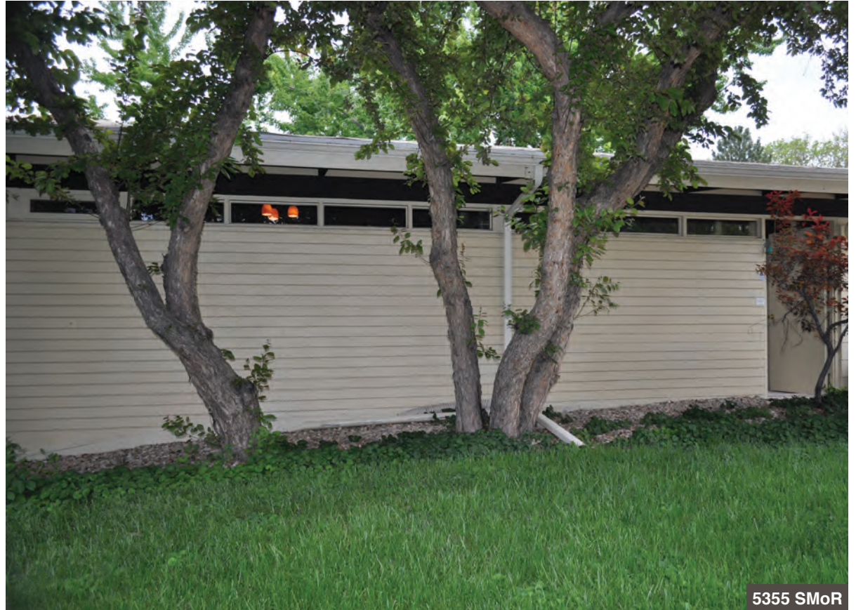
A single exterior wall extends the length of the house, across an open breezeway, and onto the face of the garage, creating the illusion of a much larger dwelling.
