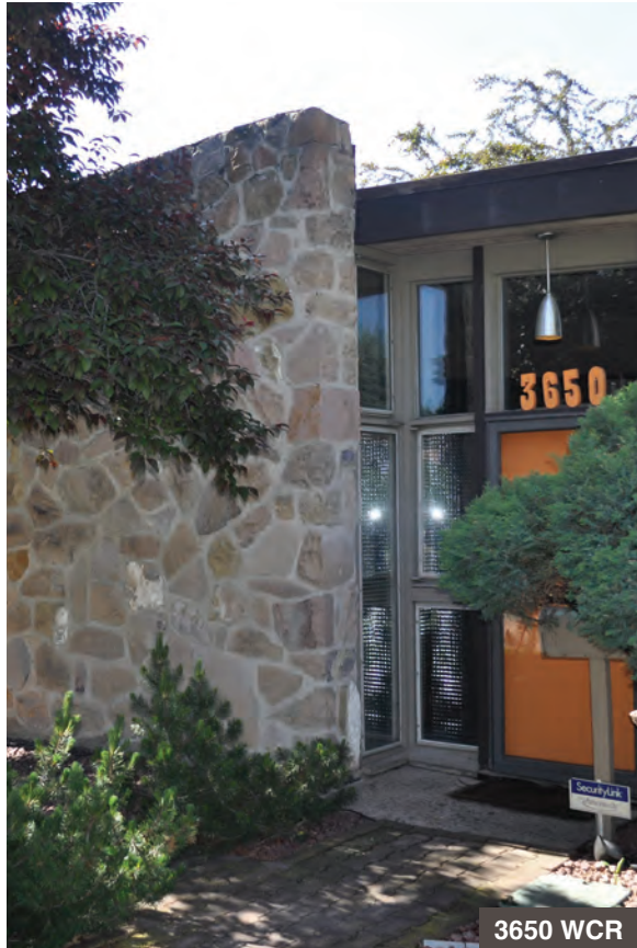
This rhyolite chimney wall sits entirely in front of the roof plane. Behind, perpendicular sidelights appear adjacent to the front entry.
