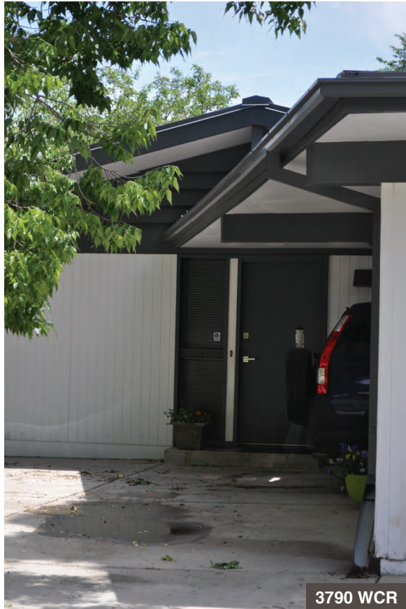
Projecting and overlapping roof and wall planes create complex compositions on many Arapaho Hills Houses.
