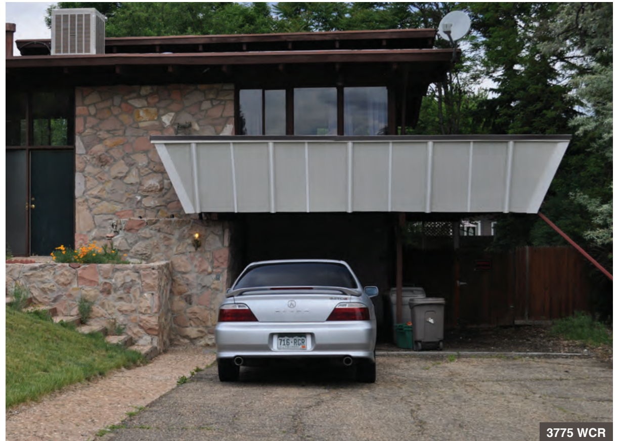
The cantilevered balcony extends around the corner of the house and terminates on the face of the chimney.
