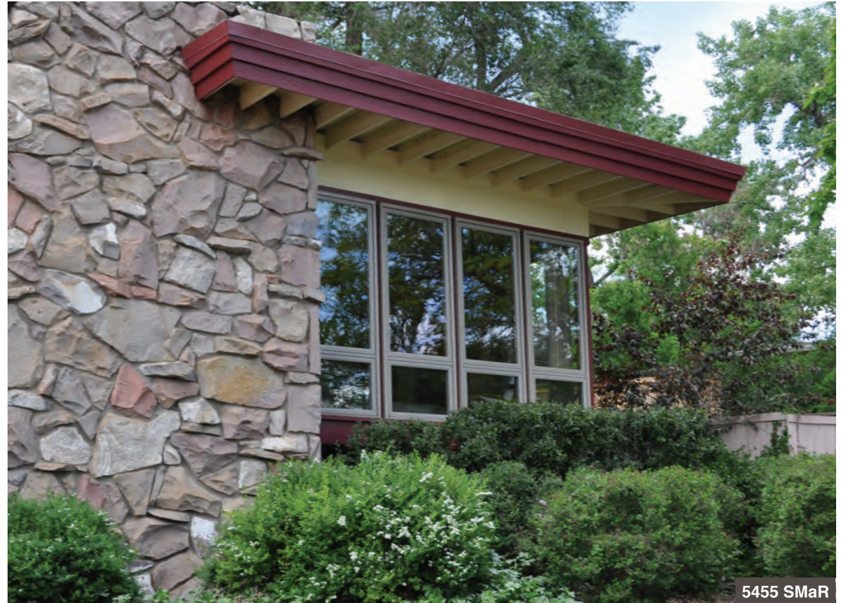
An eave composition with angled three-course lapboard fascia shelters a full-height window on the wall below. It extends onto the face of the adjacent chimney.
