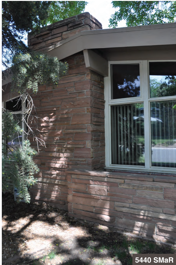
A chimney with overlapping roof fascia and planter box form defining features of this primary elevation.
