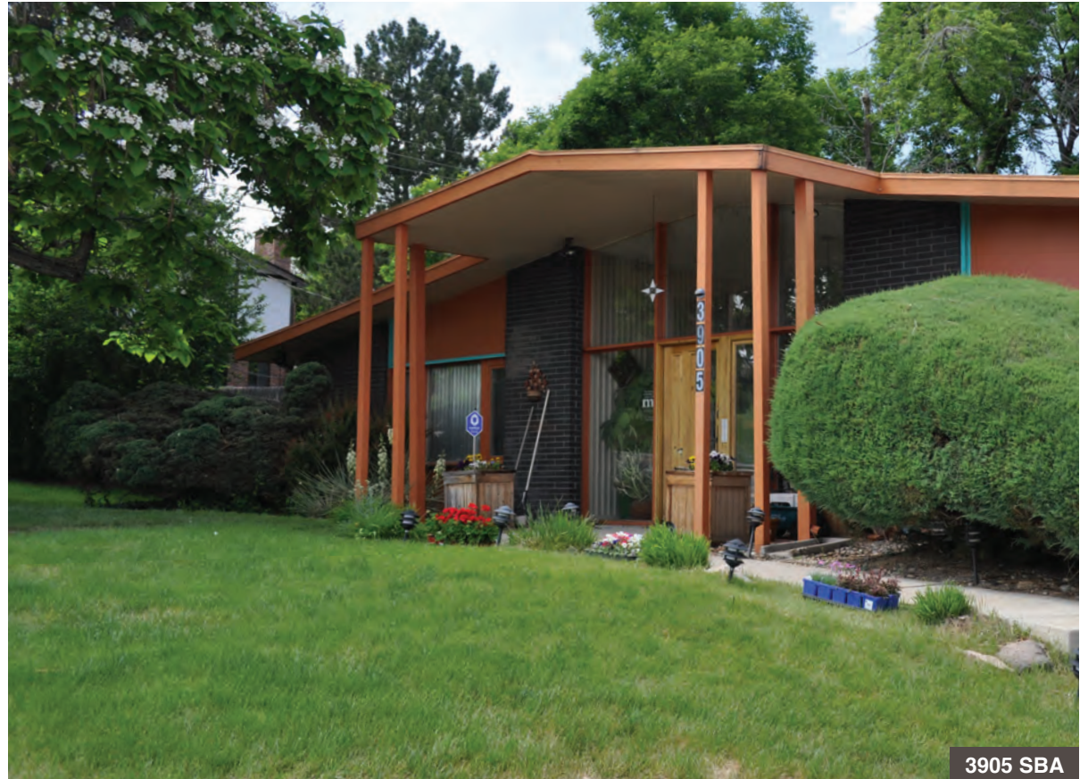
The peak of this front-gable roof projects beyond the body of the house to form a porch cover for the entrance.
