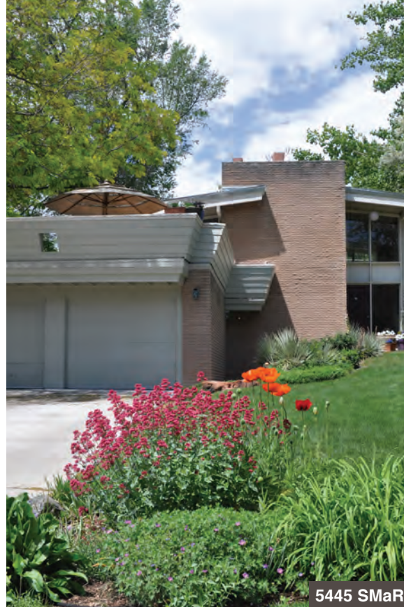
A balcony fascia atop the garage and a massive chimney define this home.
